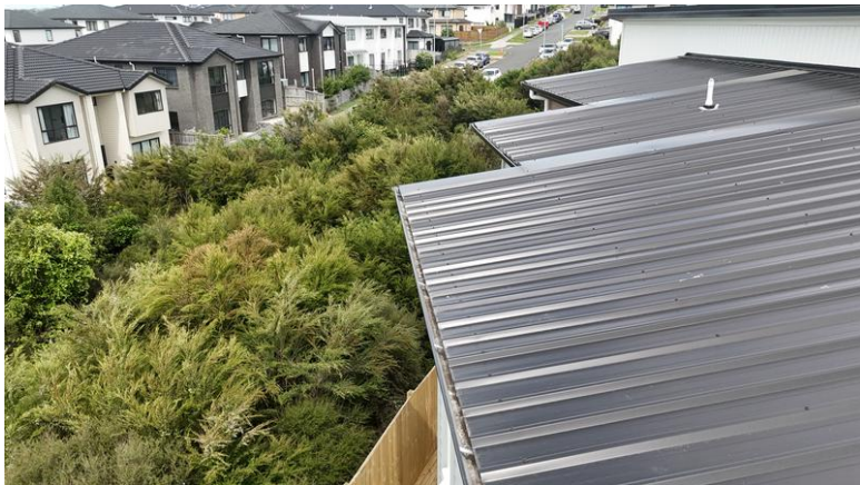
Photo 12 Gutters clear at the time of inspection.
