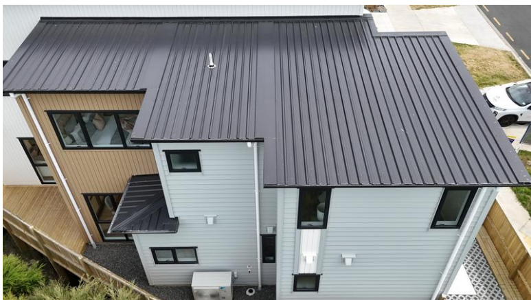
Photo 4 Profiled metal roof to the north side of the dwelling with a painted coating. No visible issues observed at the time of inspection.
