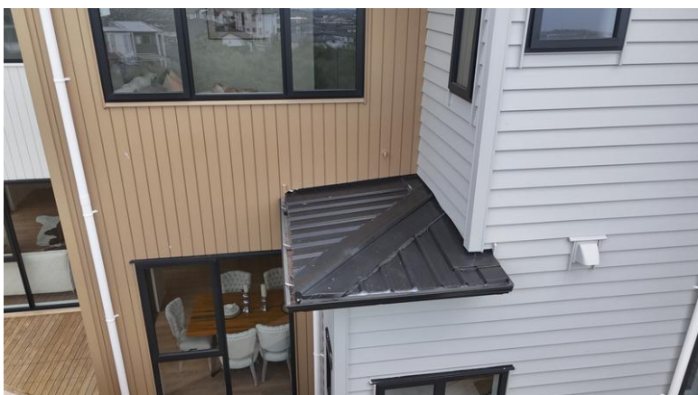
Photo 6 Profiled metal roof to the lower north side of the dwelling with a painted coating. No visible issues observed at the time of inspection.
