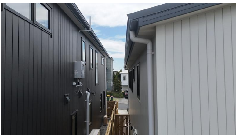
Photo 13 Profiled metal gutters connected to uPVC downpipes are installed in front of profiled metal fascia boards, with painted fibre cement soffit linings fitted beneath the eaves.
